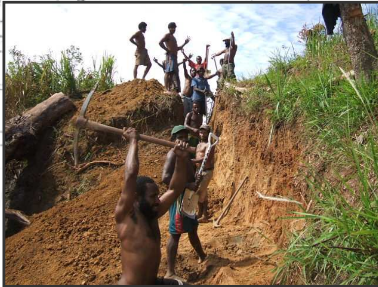
Trenching at Gossan Hill
